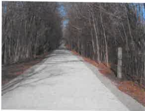
Stone dust surface, 10-foot wide
